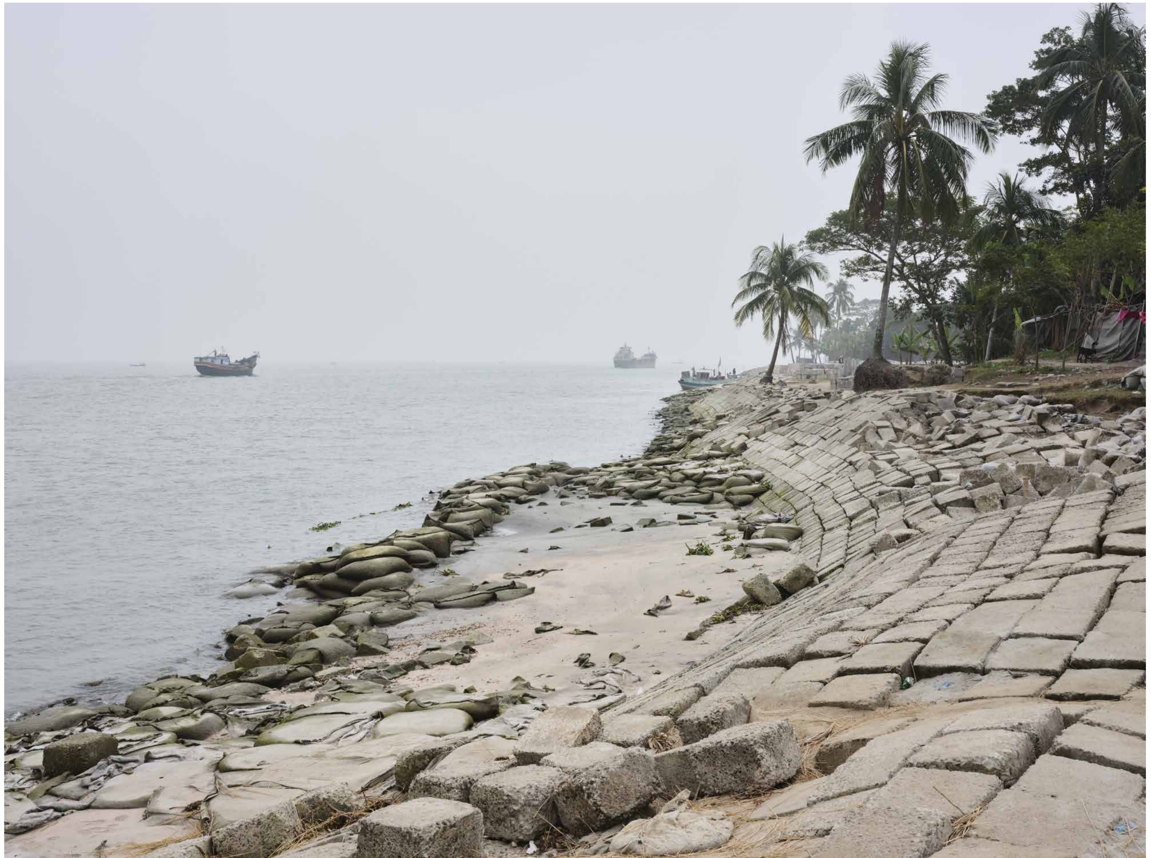
Sandbags and heavy concrete blocks are used to control the riverbank erosion. Ulania, Mehendiganj Upazila, Barisal District, Barisal Division.
