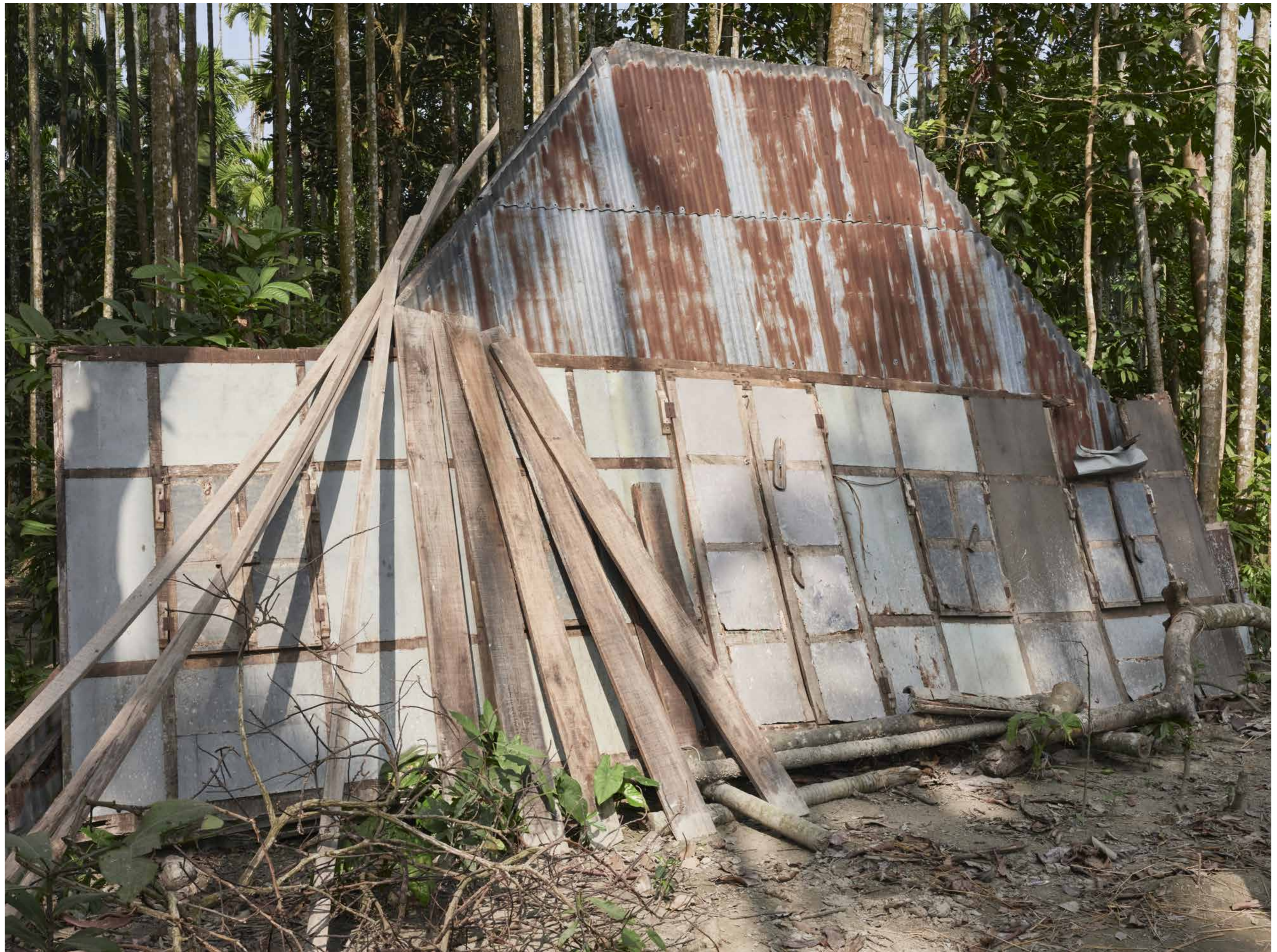
In the coastal areas of Bangladesh it is common for people to be displaced a number of times. This house was built in such a way that it can be dismantled and moved to a new location if required. Char Hogra, Mehendiganj Upazila, Barisal District, Barisal Division.
